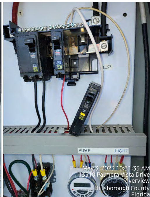
Above – the ground fault cable has been cut, turning this into a “regular” breaker. When we attempted to replace the breaker it just kept tripping. Please see proposal for necessary repairs on the following page.
