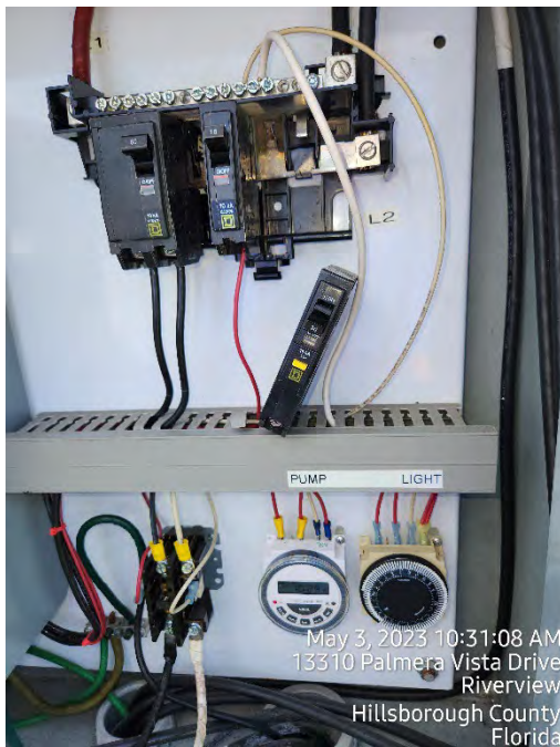
Above – the ground fault cable has been cut, turning this into a “regular” breaker. When we attempted to replace the breaker it just kept tripping. Please see proposal for necessary repairs on the following page.
